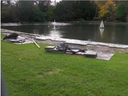
For most of the time the weather was against the workmen as can be seen from the rather damp conditions in the photographs, it would appear that attempts to create a coffer dam and repair the path from the water side, was not successful so a trench was dug behind the original path and this was filled to form a barrier. This backfilling was then paved over and the path repaired where
